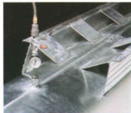
Each pontoon chamber is tested by air valves for any leaks in the weld seams.
