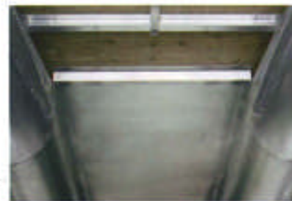
Thru-bolting is used to provide proper deck fastening and the elimination of screw heads backing off.
