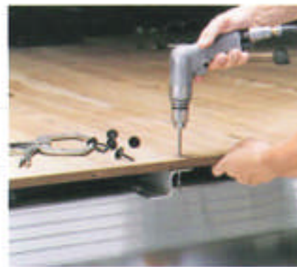
Thru-bolting is used to provide proper deck fastening and the elimination of screw heads backing off.
